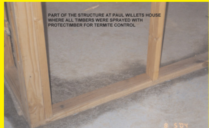
Structural timbers can be treated.
